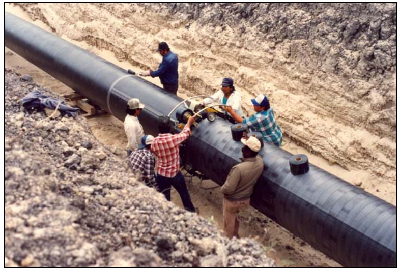
Application of RD-6 by machine is strongly recommended wherever possible. The increased tension of machine application assists in resisting soil stress.
