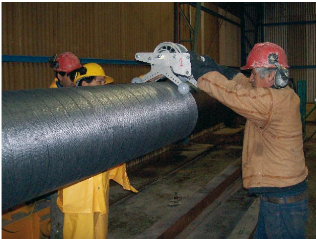
Figure 1. Plant application of Polyguard RD-6 in Chile.
